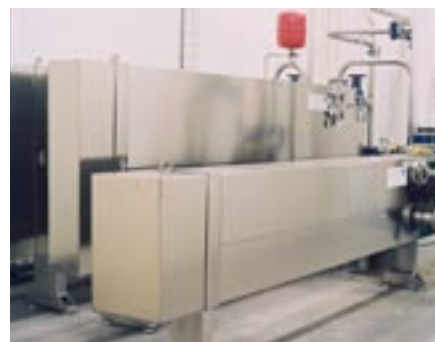
Heat exchanger sludge/water and heat exchanger unit sludge/sludge from Läckeby Products installed in Älmhult.
